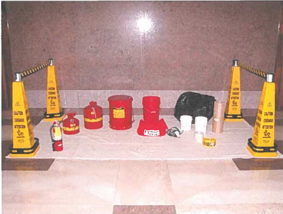
An example of using the tarp for your work site setup.
